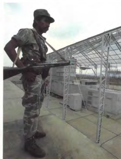
Salvadoran soldier stands guard over U.S.-funded emergency generator which helps to restore electric power when guerrilla activity disrupts normal public services.
