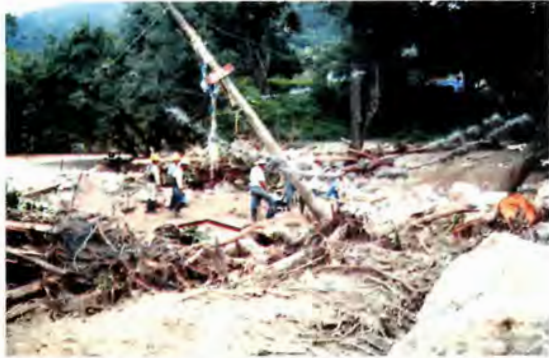
Damage to El Jicarito's electrical system.
