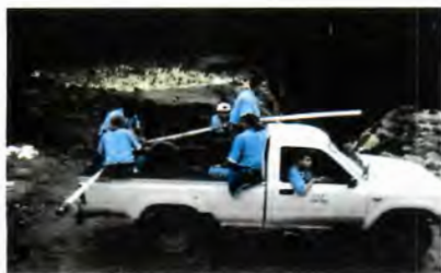
Students repairing potable water systems.
