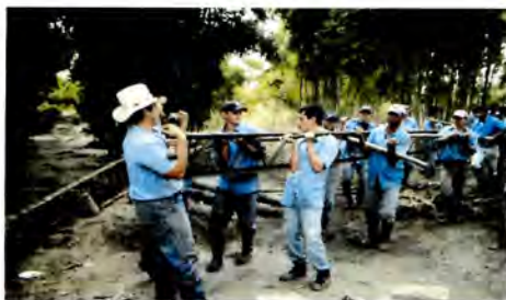
A group of students builds a bridge to connect Zamorano's potable water system.
