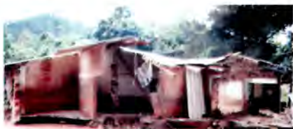
A damaged house in El Jicarito.
