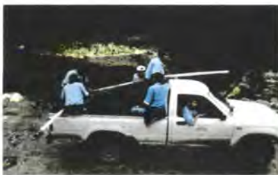
Students repairing potable water systems.
