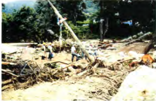
Damage to El Jicarito's electrical system.
