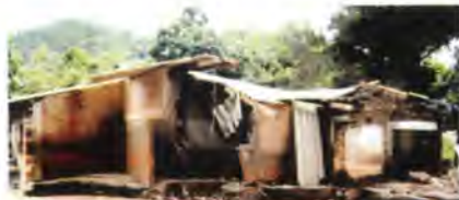
A damaged house in El Jicarito.
