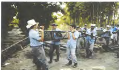
A group of students builds a bridge to connect Zamorano's potable water system.
